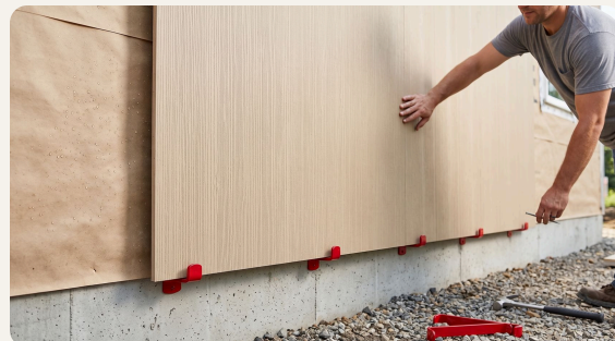
THE PANEL RESTS ON WALL-MOUNTED HOOKS. FEET VISIBLE BELOW THE BOTTOM EDGE.
